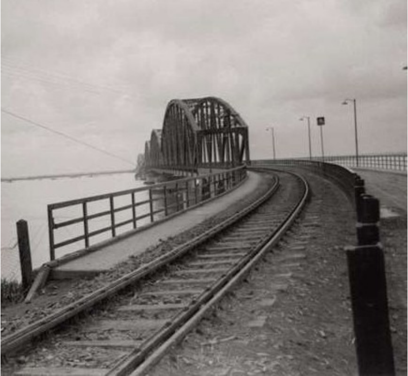
King Petar II Bridge, center spans blown
